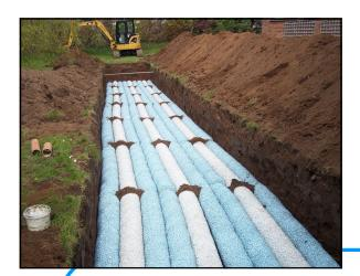
Underground soakaways are normally the preferred method of effluent dispersal in the UK but only when soil conditions are suitable for their installation.
